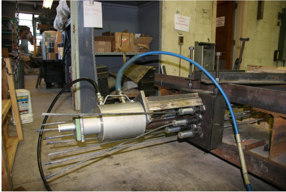
Figure 6-8. Stressing of the column strands
