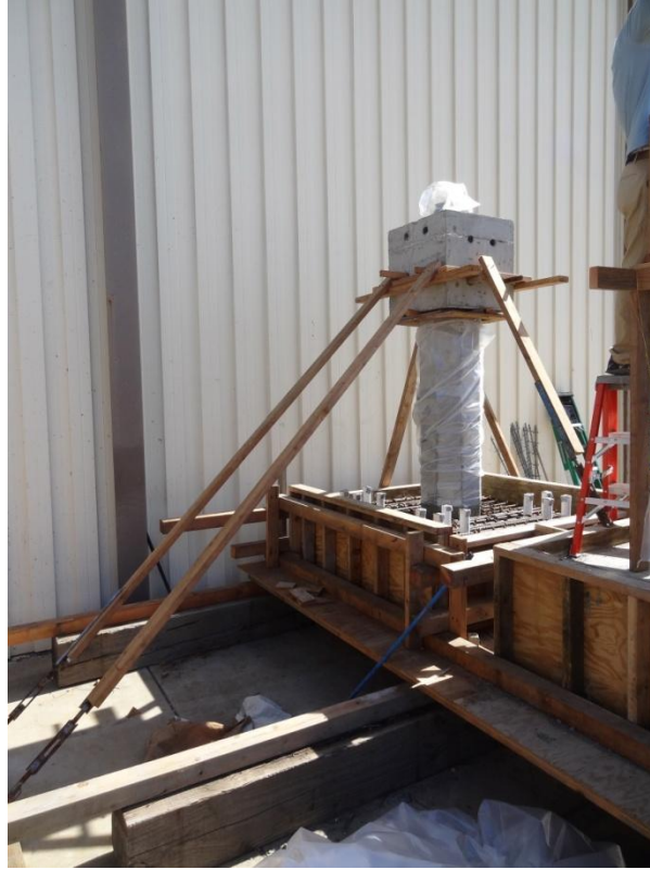
Figure 6-12. Specimen PreT-SF-FIB-SHK braced and ready for casting of the foundation
