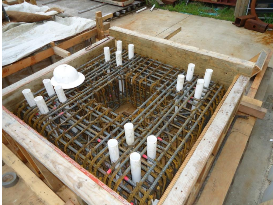
Figure 6-10. Spread footing ready for installment of Specimen PreT-SF-FIB-SHK
