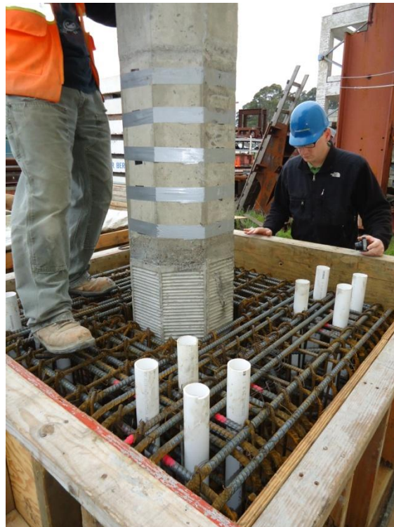
Figure 6-11. Specimen PreT-SF-FIB-SHK being lowered into the foundation
