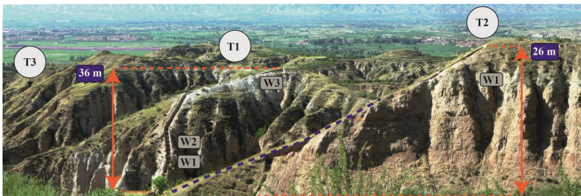
Figure 7.2 Exposed sediment sections T1 to T3, including white marker layers W1, W2 and W3. The thicknesses of T1 and T2 are indicated and the dividing Youfang Fault (broken blue line) which caused a vertical displacement of approximately 30 m. The Sanggan River is flowing in the valley located N of the sampling locations (in the background)
