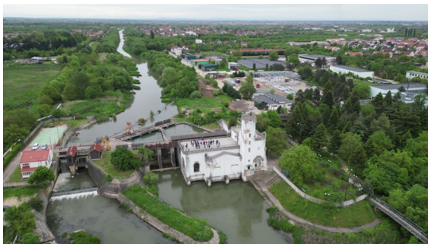
Fig. 29 Aerial view of the Timișoara SHPP (from downstream)
