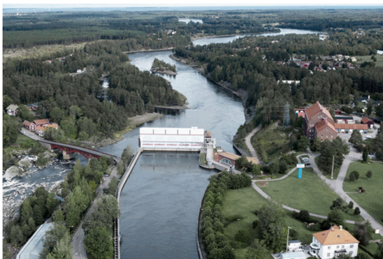
Fig. 63 Old and new Älvkarleby hydropower plants: aerial view (in flow direction)
