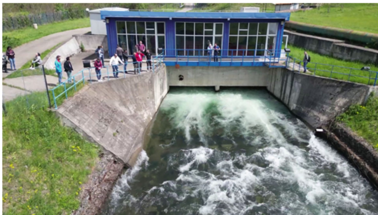
Fig. 27 Zervești SHPP surface power house and tailrace channel (view from downstream)
