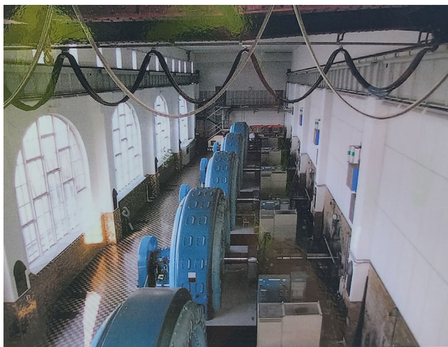
Fig. 65 Old Älvkarleby machine hall equipped with five horizontal hydropower units commissioned in 1915
