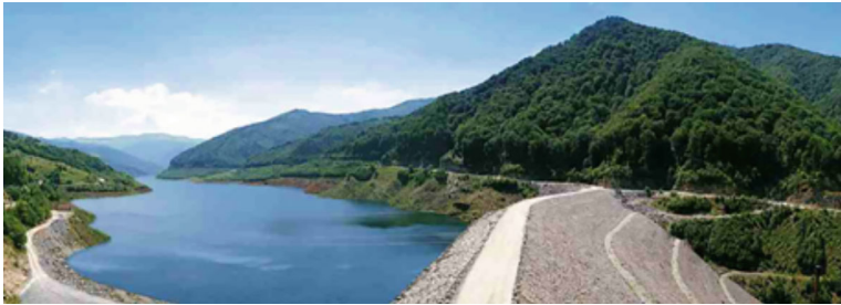
Fig. 21 Poiana Mărului reservoir view and Măru concrete faced rock-fill dam with clay core [43]
