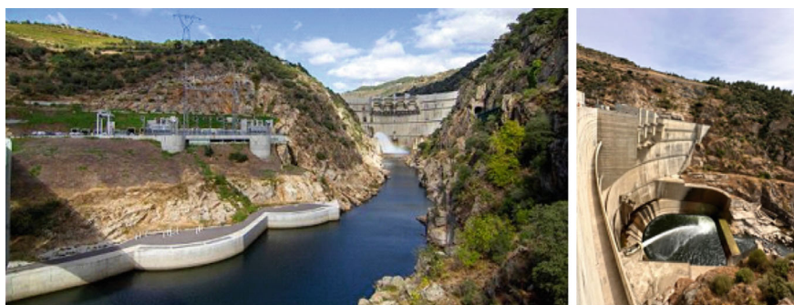
Fig. 57 Foz Tua pumped storage hydropower plant (PSHP); a Downstream view, and b right bank view [14]
