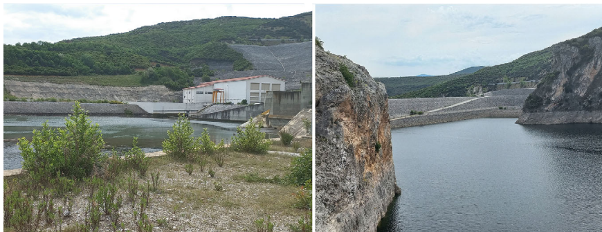
Fig. 48 The Ilarion dam (downstream and upstream view)
