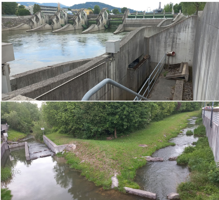
Fig. 72 View of the two type of the fish passage systems installed at the Sohlstufe Lehen RoR HPP
