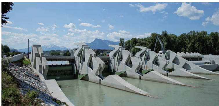
Fig. 71 Sohlstufe Lehen RoR HPP (view from downstream) [46, 49]
