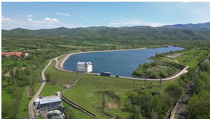
Fig. 25 Aerial view of the Zervești hydropower system
