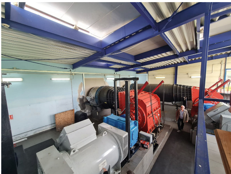
Fig. 26 Zervești SHPP machine hall equipped with two HPU's
