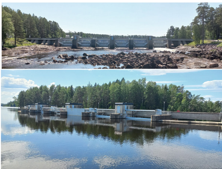
Fig. 66 Älvkarleby spillway and dam
