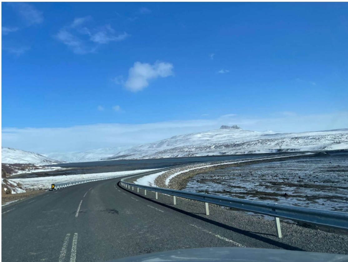
Figure 32 The new road across one of the fjords in the Teigsskógur area. Image: EBE.
