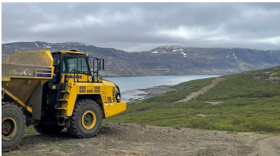
Figure 35 Overlooking Teigsskógur scrub and the new roadbed in June 2022. Image: EBE.
