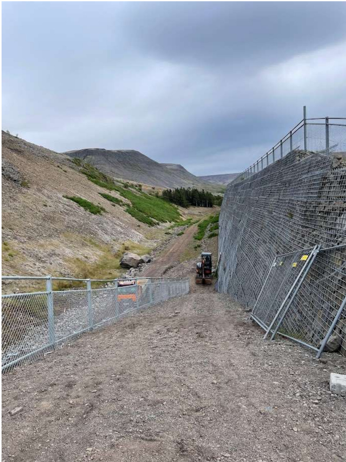
Figure 15 On the avalanche fences, which are a wall made from the mountain itself, a relocated mountain is in front of the mountain to shelter the human community beneath. Image: EBE.
