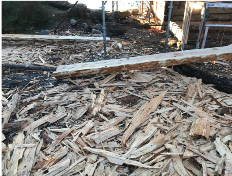
Figure 66. Woodworking in Sunnmøre Museum, Norway. Traditional Norwegian log houses were being renovated for which the carpenters' used axes, commonly used between 1100-1400; note the amount of debris (Photo: Lisabet Guðmundsdóttir).
