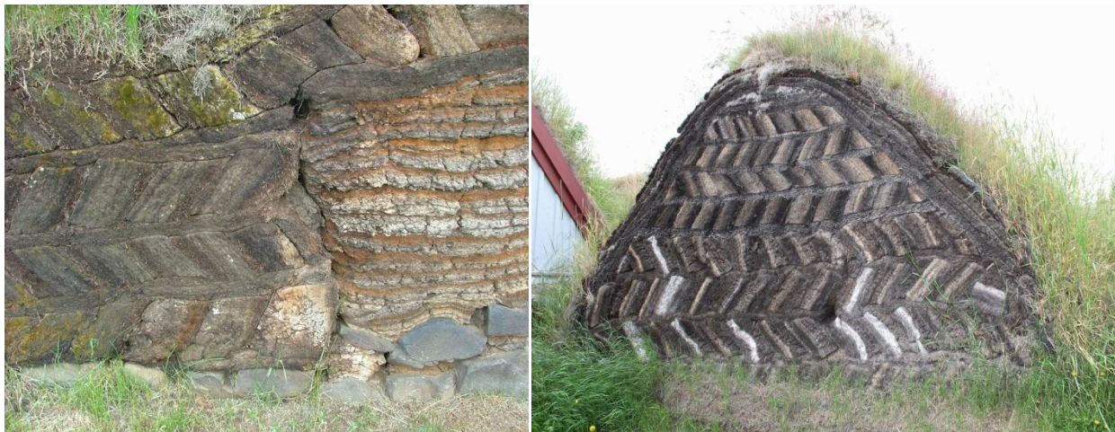
Figure 3.1: Strengur and klambra blocks stacked together to form wall at Glaumbær farmstead (left), and klambra wall at Laufás farm (right).
