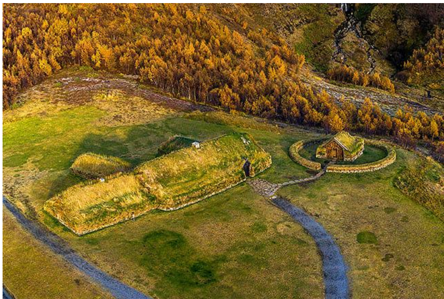
Figure 3.6: Aerial view of Stöng (Source Iceland360vr).
