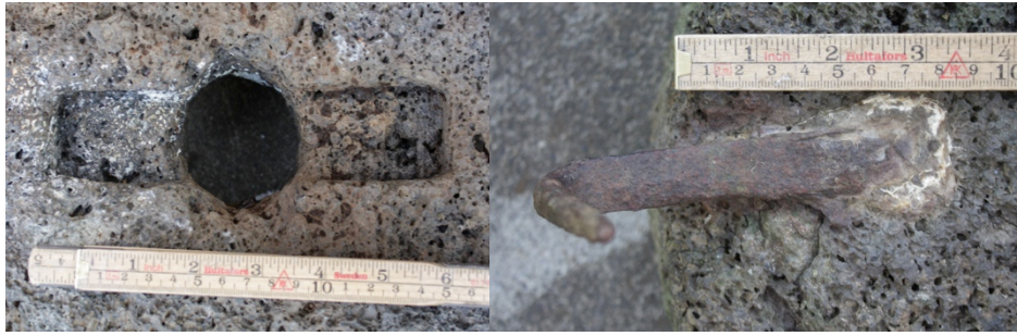
Figure 6.32. Stóra-Sandfell in Skriðdalur (221), larger and rectangular oblong rynd slot and an angled iron handle in socket fused with tin (or lead).
