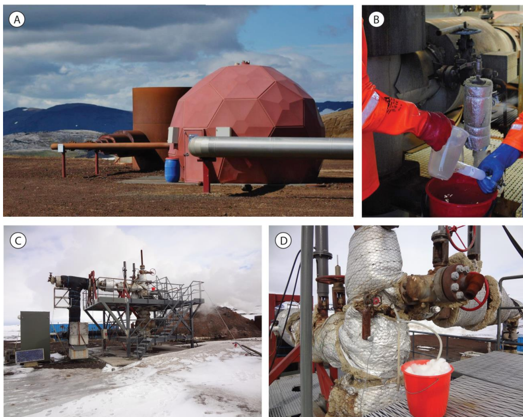
Figure 4 Two-phase geothermal wells in the Krafla geothermal field (A) and (B); (C) the IDDP-1 well; D) close-up image of the sampling setup (images are courtesy of Nicole Keller).
