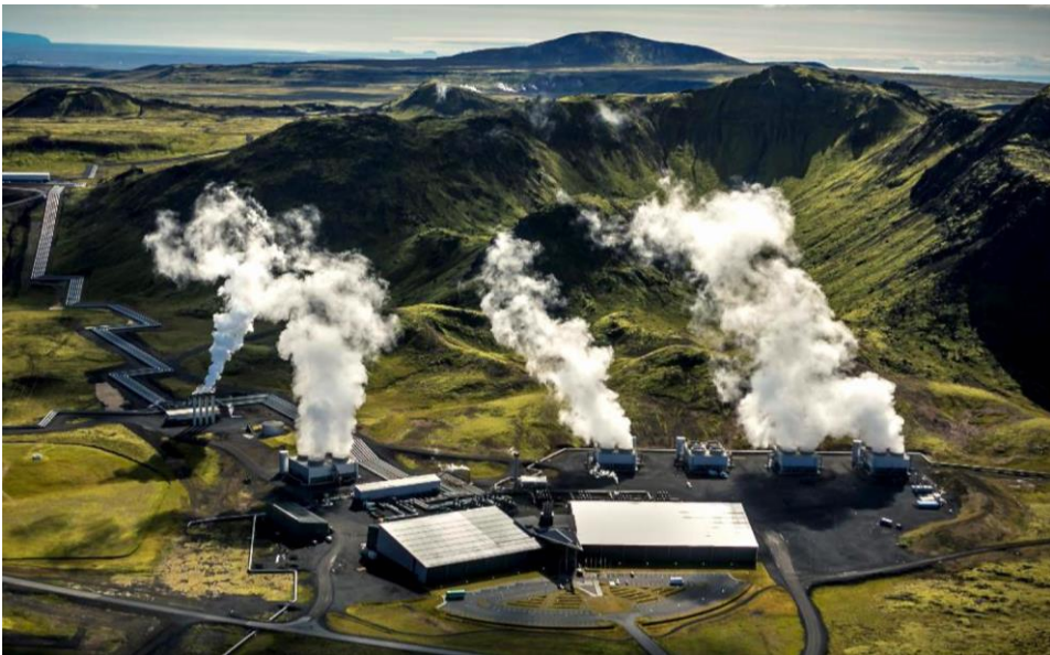
Figure 1.2. Hellisheidi geothermal power plant in subarctic Iceland. The area is dominated by the Racomitrium lanuginosum (Hedw.) Brid., moss plants (Photo: Reykjavik Energy, 2016).
